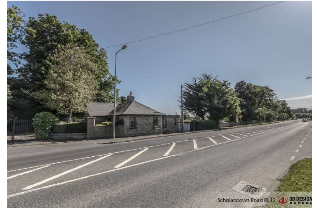
C - Adjacent gate lodge to south east of site
